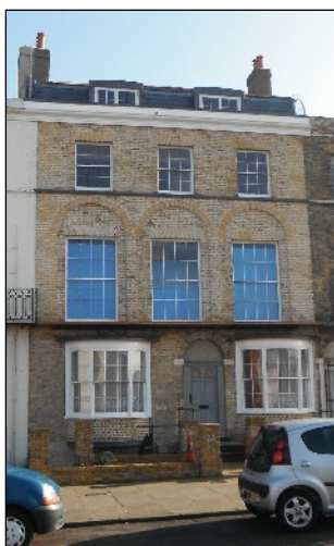
12 Zion Place, Cliftonville (Renovation)
