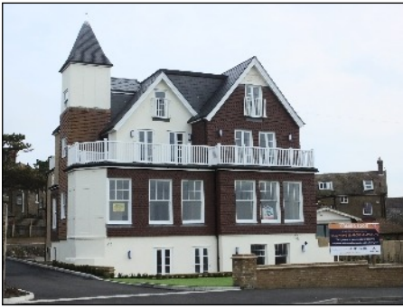
April House, 69 Sea Road, Westgate-on-Sea (Conversion to eight apartments)
