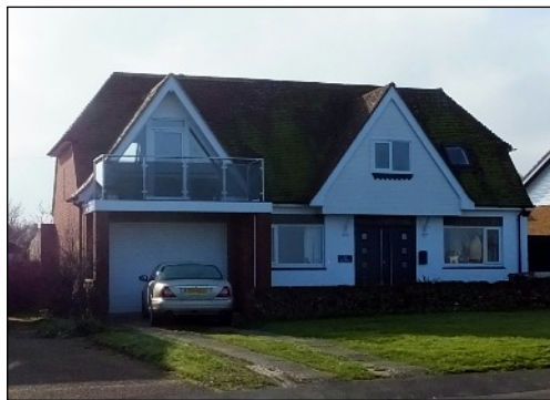
Beside the C, 131 Sea Road, Westgate-on-Sea (Extension to property)
